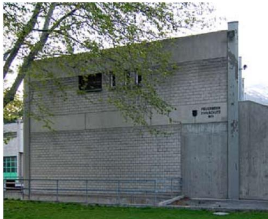
The masonry gable wall strengthened by vertical CFRP-strips.
