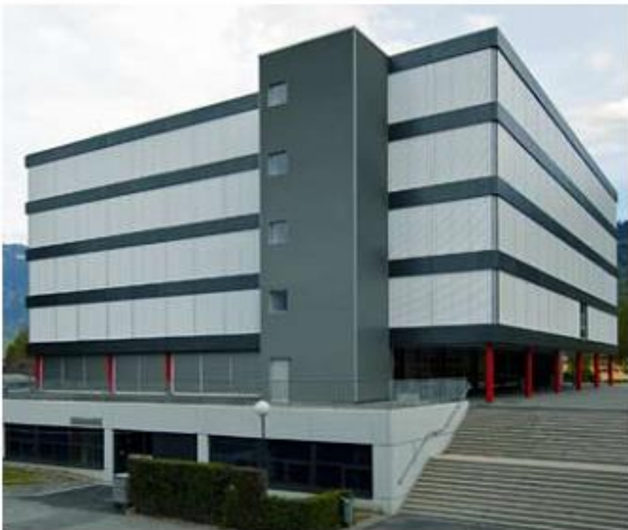
View of the new stairway tower on the north side of the building.
