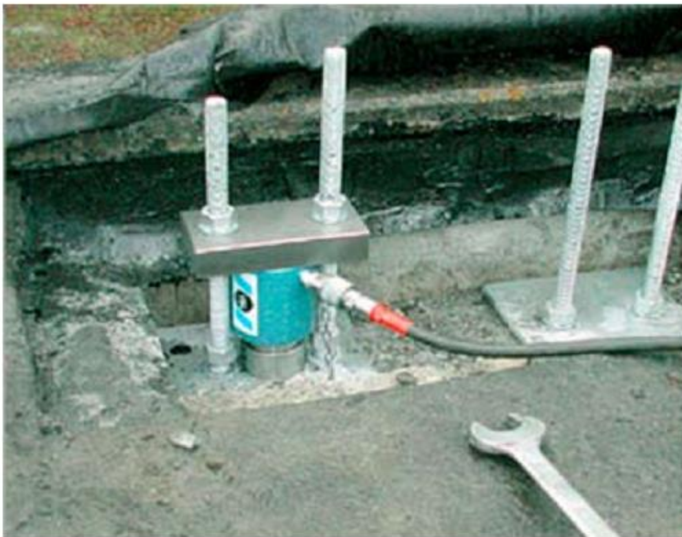
CFRP-strips post-tensioned from the roof (Truffer et al. 2004).
