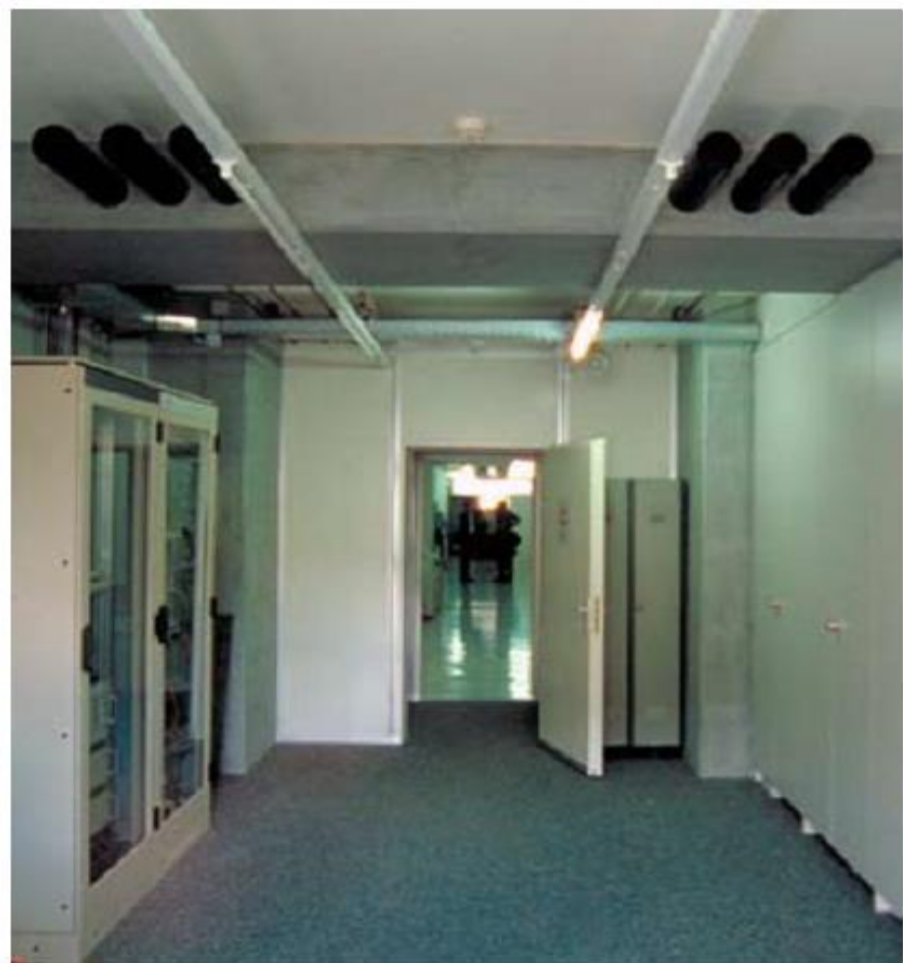
View of the 6 anchorages of the tension strands in the cross girders between both new I-shaped reinforced concrete walls in the extension.
