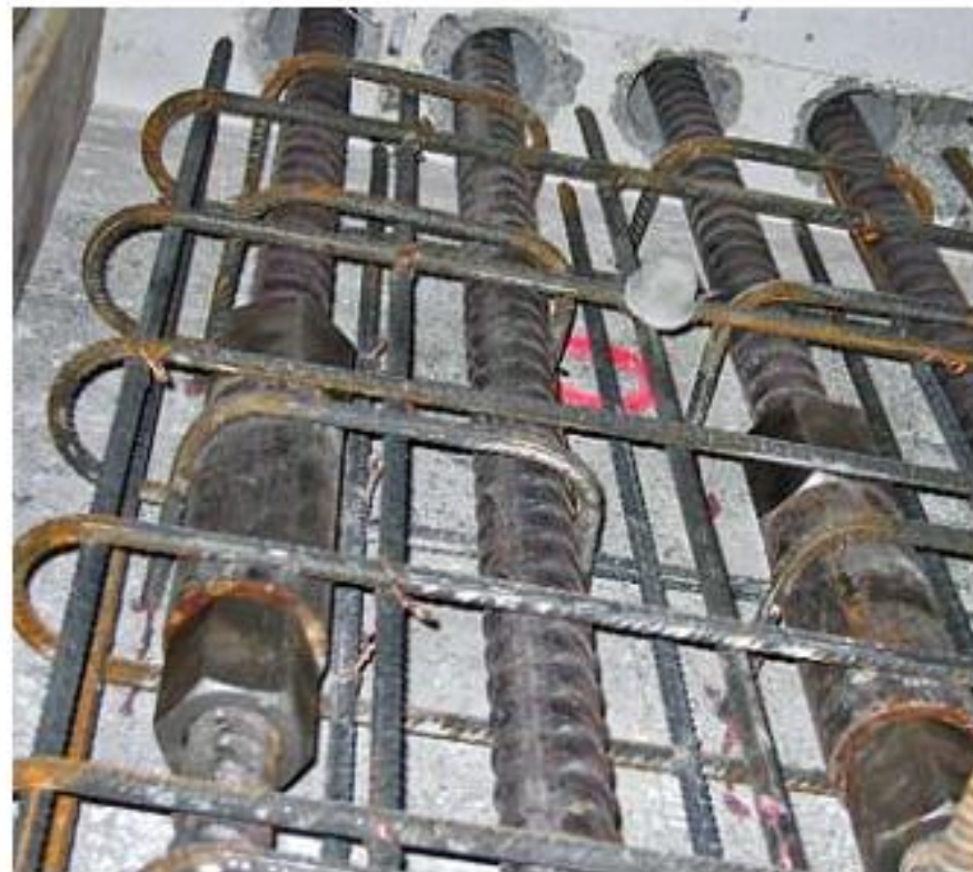
Detail of the vertical reinforcement couplers in the double wall.
