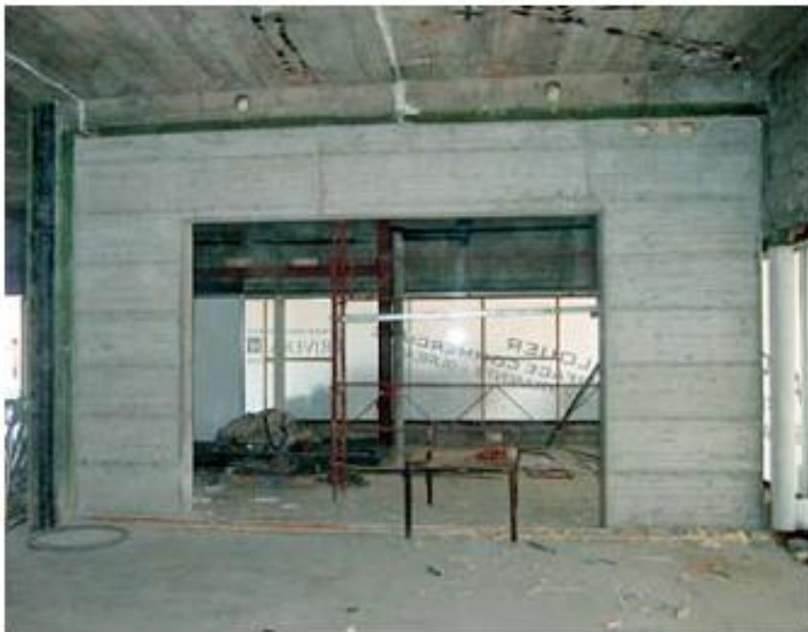
New reinforced concrete frame in the ground floor level.
