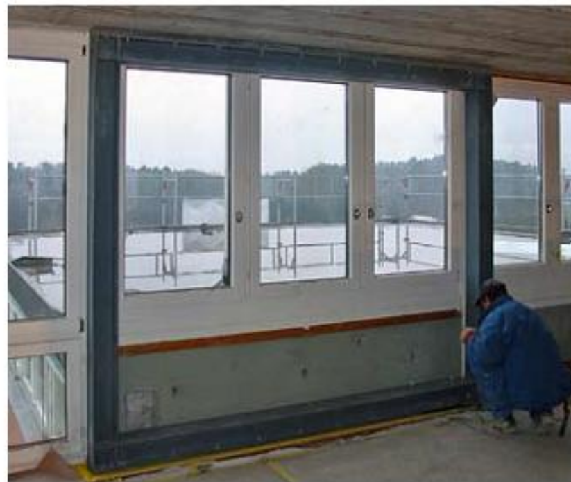
Bracing the roof level with new steel frames.
