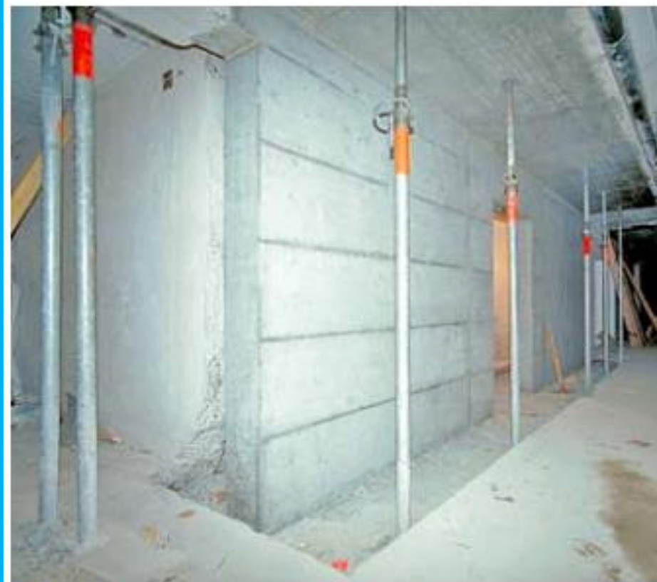
New coupled reinforced concrete structural walls in the basement.
