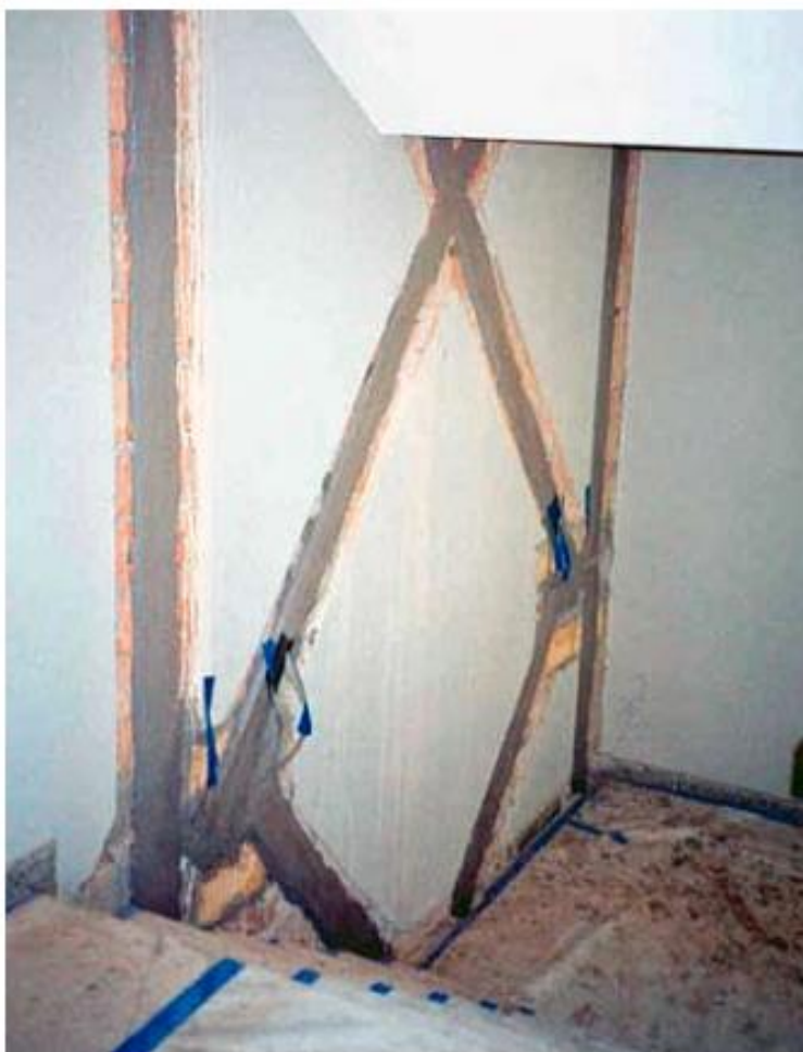
Strengthening of the masonry walls in the staircase with CFRP-strips.
