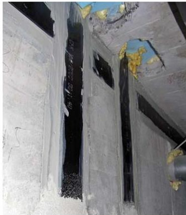
Strengthening of the elevator shafts with bonded carbon fiber strips.
