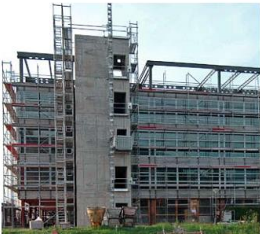
Stairway tower and addition under construction (south side).
