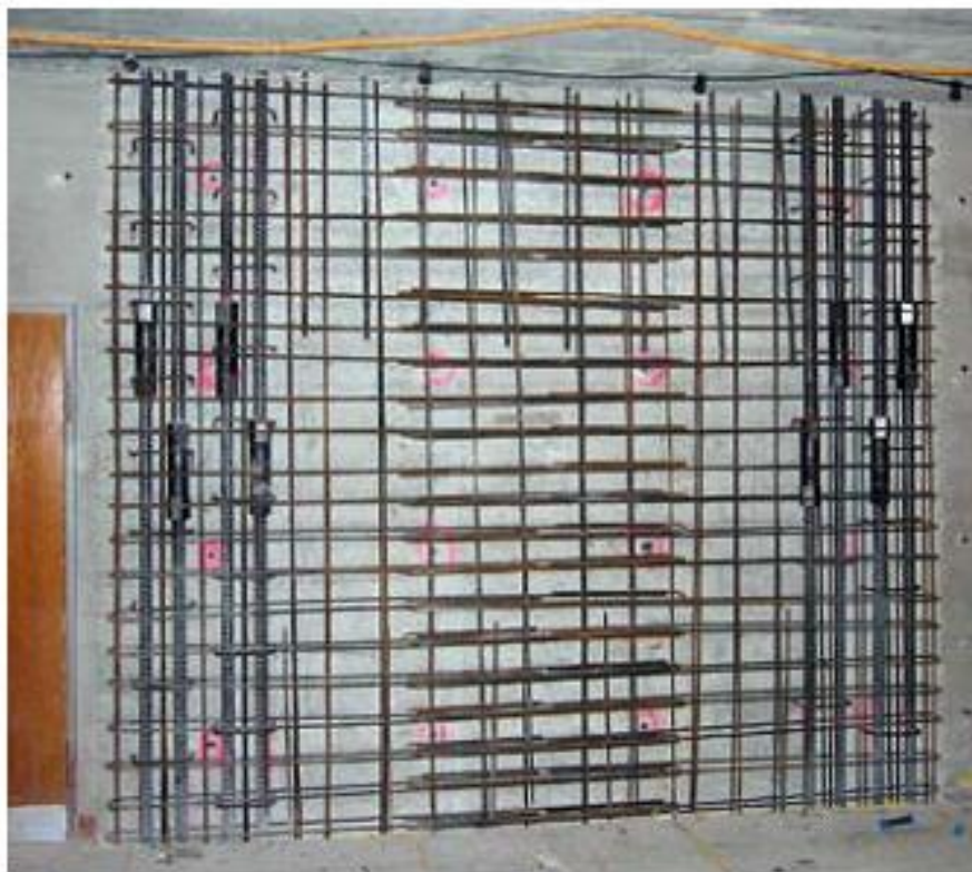
Reinforcement in the composite wall with vertical reinforcement couplers.
