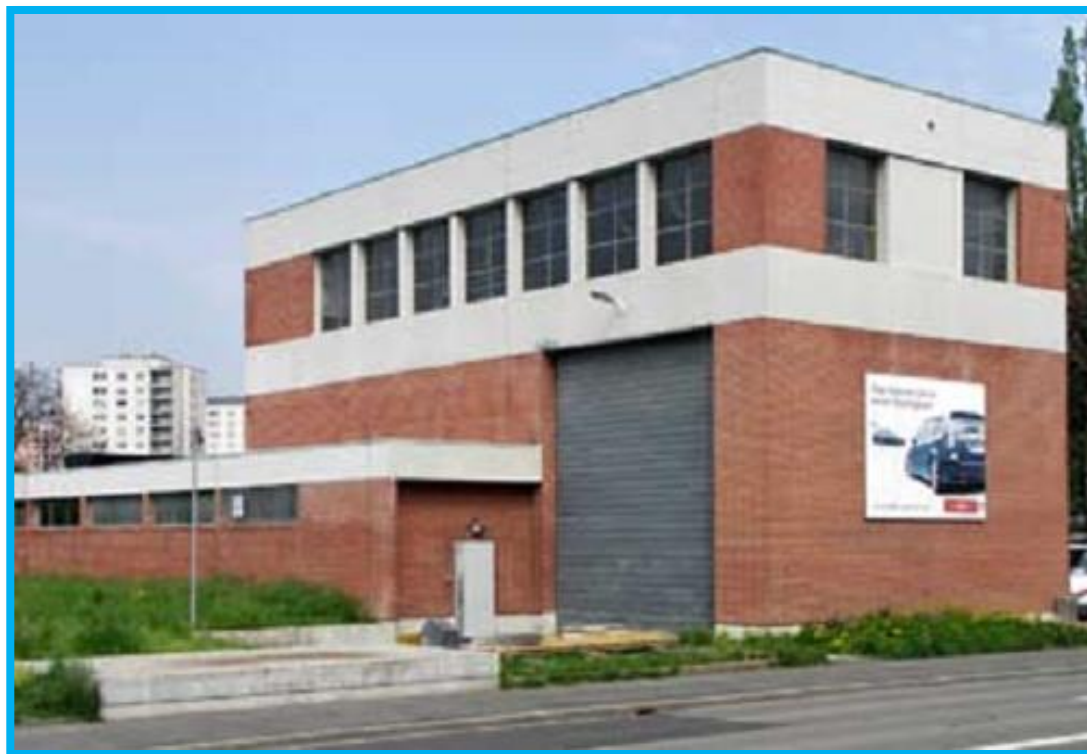
Substation in Basel
