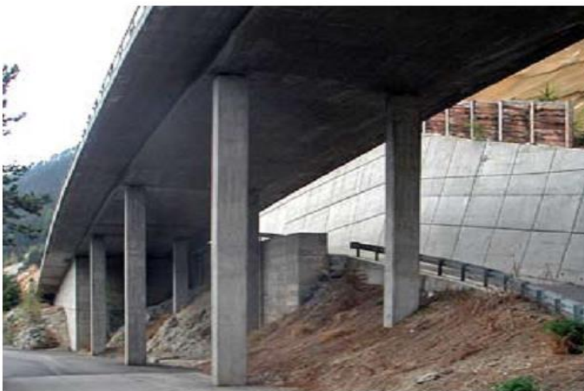
View of a portion of the bridge with tall slender columns.
