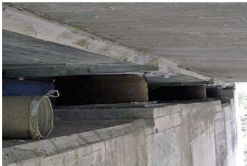
Seismic retrofit with high damping rubber bearings at the abutment.
