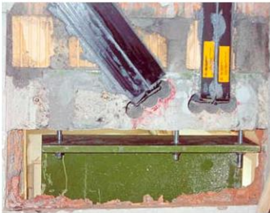
Anchorage of the CFRP-strips with shear angles in the concrete decks.
